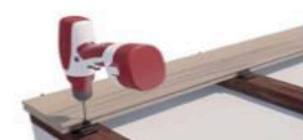
05 The fifth step Install screws
